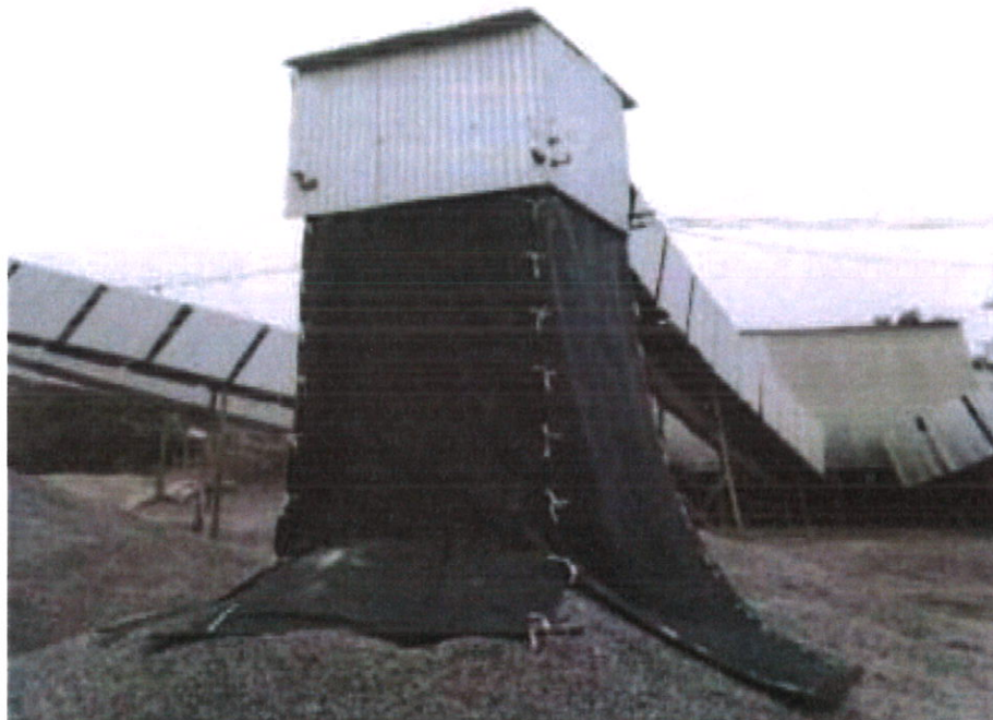
Figure-2: Chute from top of discharge point
